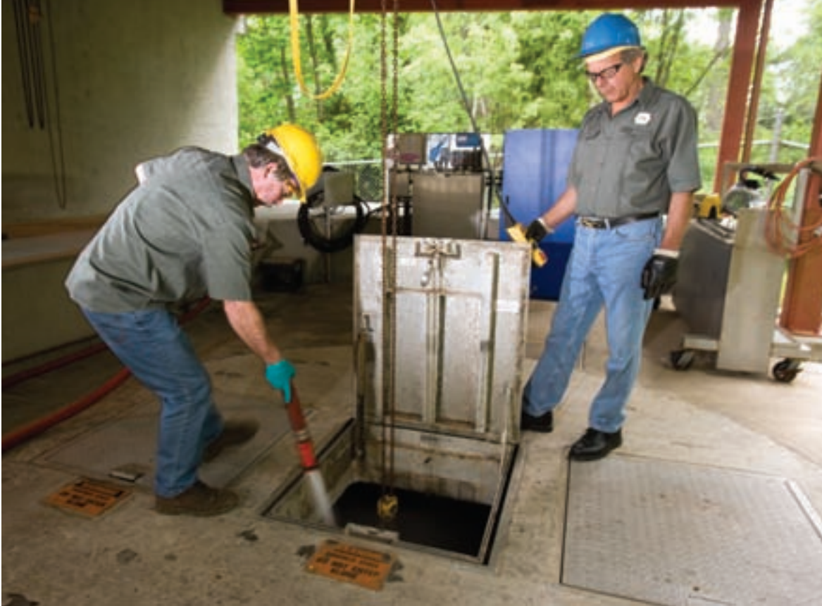
Operator Mickey Durham, left, and lead operator Don Johnson, wash down a pump at the influent pump station before pulling the pump for inspection.
